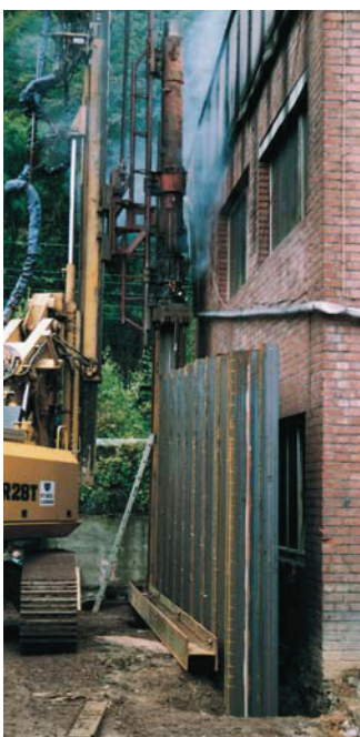
Redevelopment Altlast, Brohl-Lützing
